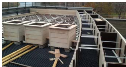
To improve aeration within the planters their inner walls have been equipped with Floradrain® FD 25-E.
